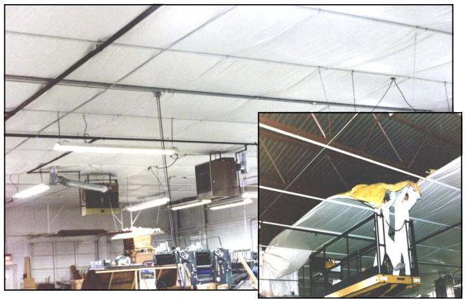
Commercial Building & Retrofit, Inc. manufactures and installs energy saving insulation systems for all types of buildings including bar joist. Compton Printing Inc. insulated this 15,000 sq.ft. facility and turned it into an energy efficient building reducing the heating bill by 60%.
